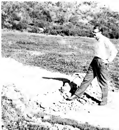
Photo 3. Fault scarp about 0.4 m high across dirt road in a farm field. One of a series of five parallel scarps with total vertical motion of about 0.8 m north of Van Nuys Boulevard along the foot of the hills. View to north. No lateral displacement.
